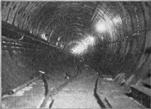
FIG. 367. — Interior of a Ten-foot Intake Water Tunnel.
